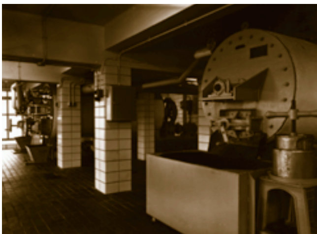
▲ Technical infrastructure : autoclave and steam production unit (1962)
