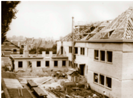
▲ Construction of building D "Foot-and-mouth disease" in 1951
