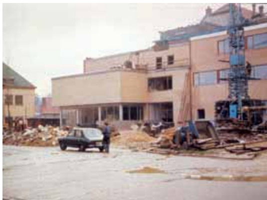
▲ Construction of building E "Virology" in 1975
