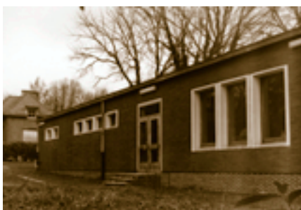
▲ The library building of the ICR (1972)
